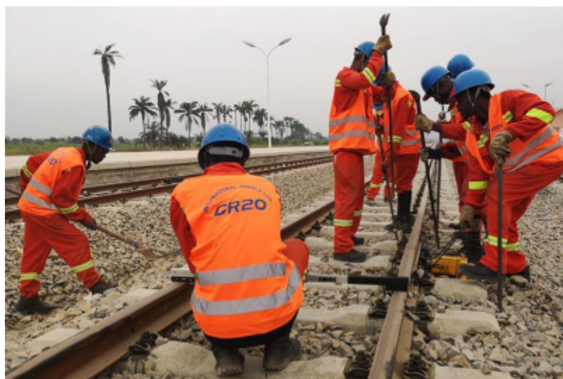
Maintenance workers, Benguela railway
